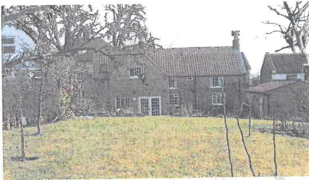
d. The rear of Lodge Cottage seen from the proposed site.
